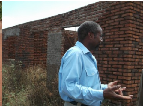
Nicholas at the Brickworks in 2013
