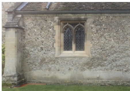
South aisle: C13 Fieldstone/flint rubble wall with Barnack in the buttress and as very large blocks in the plinth. Window restored 1866, possibly Casterton
